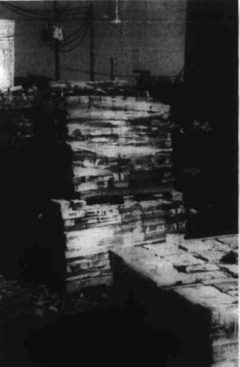
Bricks recycled What was once an imposing brick building in Eagle Lake has been reduced to rubble. The old Schumacher Building behind First National Bank was torn down last year, however, that's not the end of the story. The bricks from the building were salvaged for reuse by a company out of Houston. The pallets of brick pictured above were moved to Houston where they will begin a new life as part of another building. The Eagle Lake site is no more than a pile of rubble that seems to be creeping out into the roadway a little more each day. Headlight Photo
